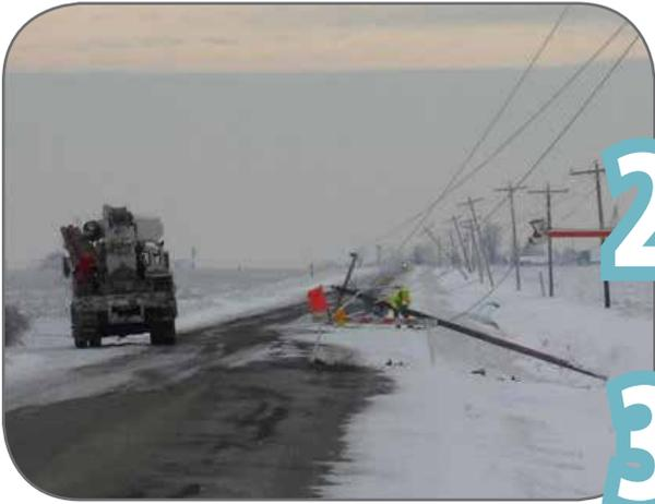
**1** **The most common cause of galloping lines is ice that builds up on one side of a power line as a result of strong winds.** This buildup creates an airfoil, which changes the flow of air around the normally round line. This change in air flow can cause the power line to start to bounce. These lines can bounce and buck so much they hit other lines, damaging themselves enough to cause a power outage or even fall to the ground.
