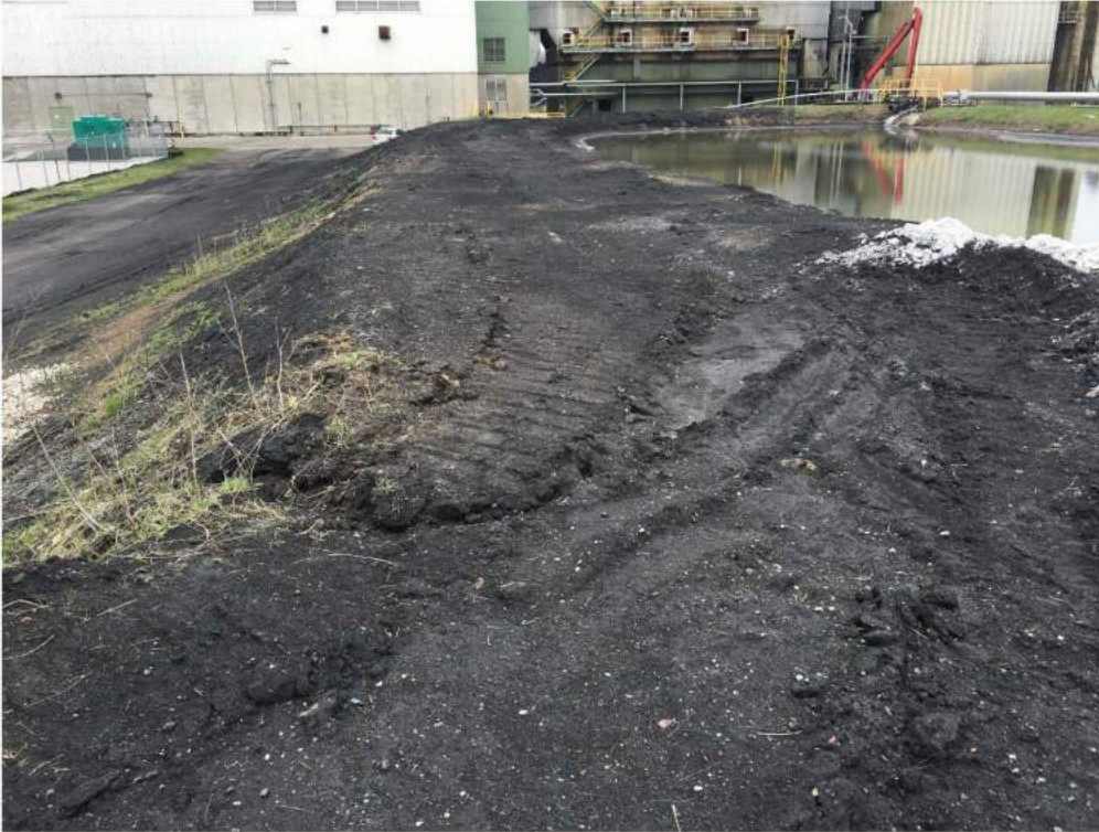
Photograph #1: East berm of the east embankment. Vegetating the exterior slope is recommended. The view is to the south. (Grand Haven Board of Light & Power, Ash Impoundments, Grand Haven, Michigan, June, 2016)
