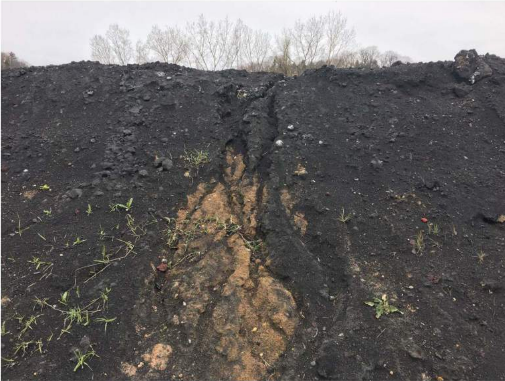
Photograph #2: Typical erosion gully on the exterior face of the east berm of the east embankment. Vegetating the exterior slope is recommended. The view is to the west. (Grand Haven Board of Light & Power, Ash Impoundments, Grand Haven, Michigan, June, 2016)
