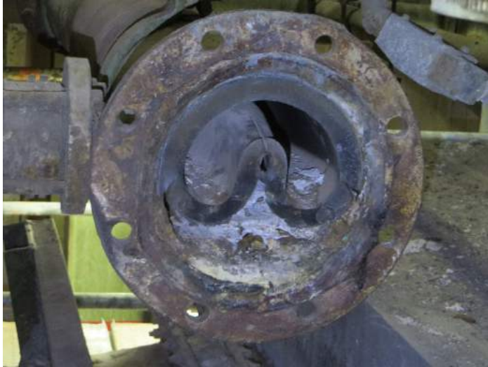
Figure 3-10 Photo of Scrubber Recirculation Pipe Liner Separation
