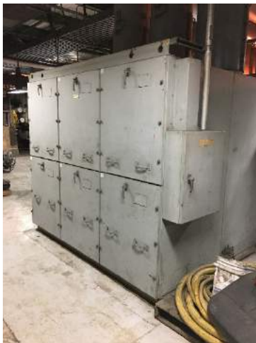
Figure 3-3 Photo of Generator PT Cabinet
