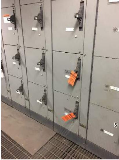
Figure 3-2 Photo of MCC Panel with Do Not Use Tags (Orange)
