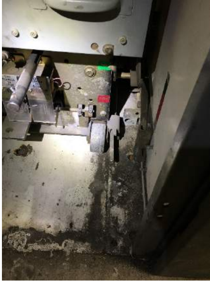
Figure 3-1 Photo of 4160V Breaker Cubical Deterioration
