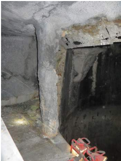
Figure 3-8 Photo of Degraded Coating and Flue Gas Deflector
