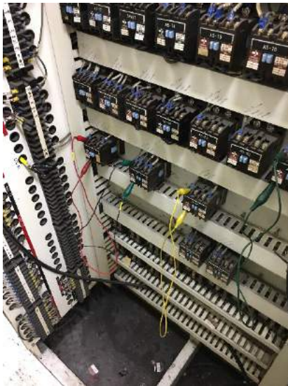
Figure 3-6 Photo of Relays with Jumpers
