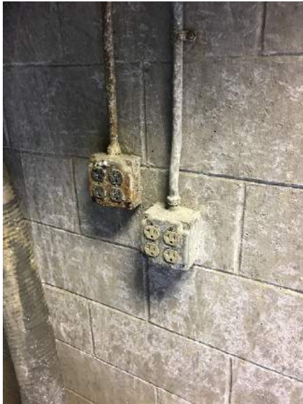
Figure 3-4 Photo of Corroded Receptacles
