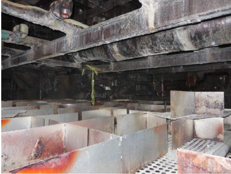
Figure 3-9 Photo of Degraded Internal Scrubber Piping
