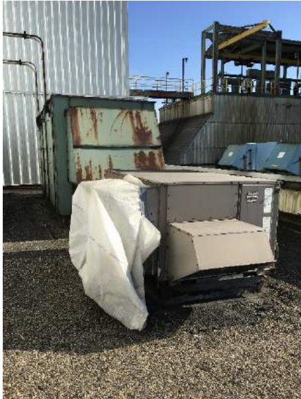
Figure 3-11 Photo of Scrubber Control Room Roof with Two Handler Units
