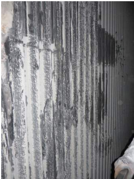
Figure 3-5 Photo of Boiler Tubes with Weld Overlay to Extend Life
