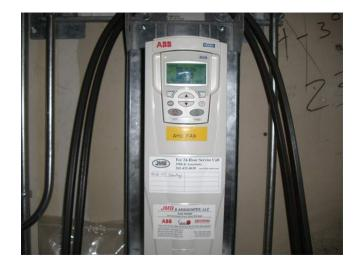
your equipment, increase productivity and minimize the costs required to maintain it. Because the equipment will run at less than its maximum speed, wear can be reduced significantly and time between routine maintenance can be extended.
