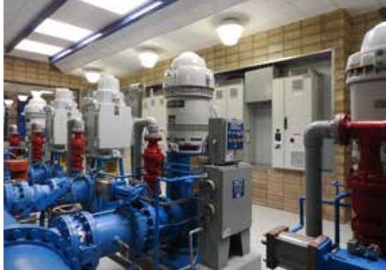
New VFDs installed on water treatment pumps to reduce energy consumption.
