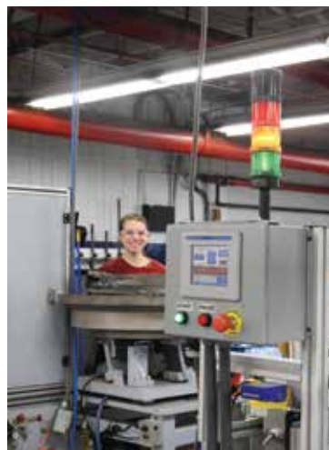
New LED lighting installed at Automatic Spring Product's Taylor Avenue facility.
