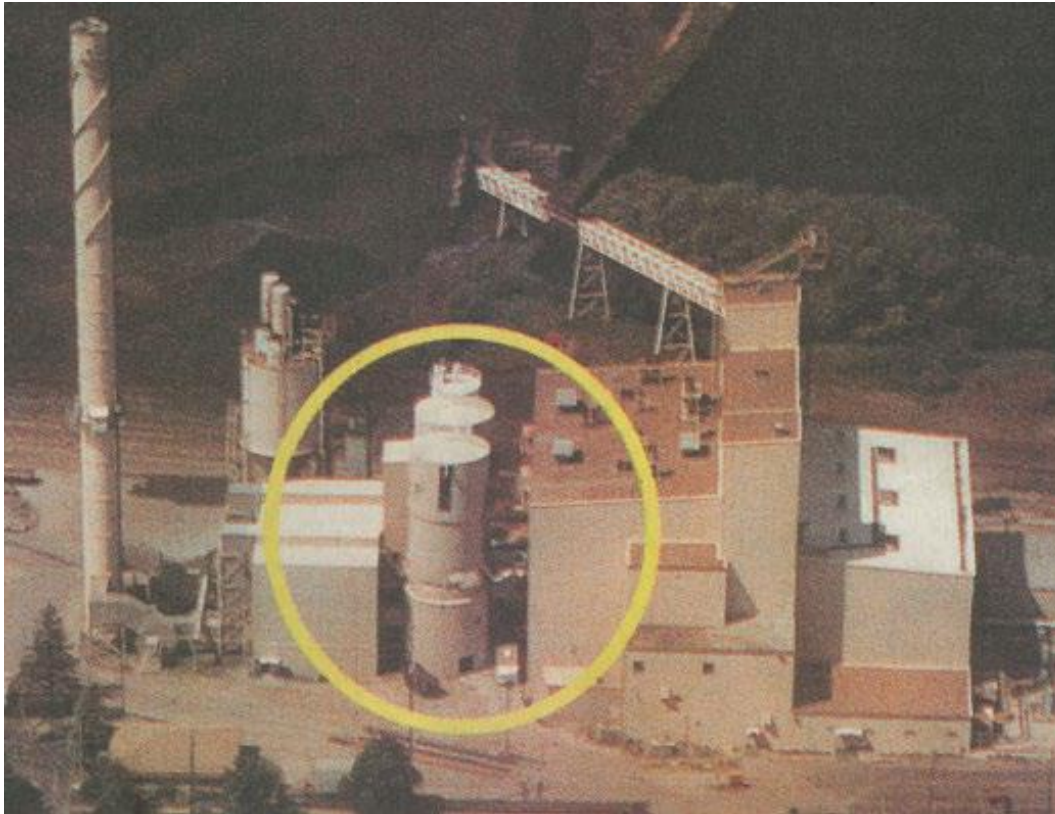
T.E.S Filer City Manistee, MI Scrubber Vessel Failure (2002)
