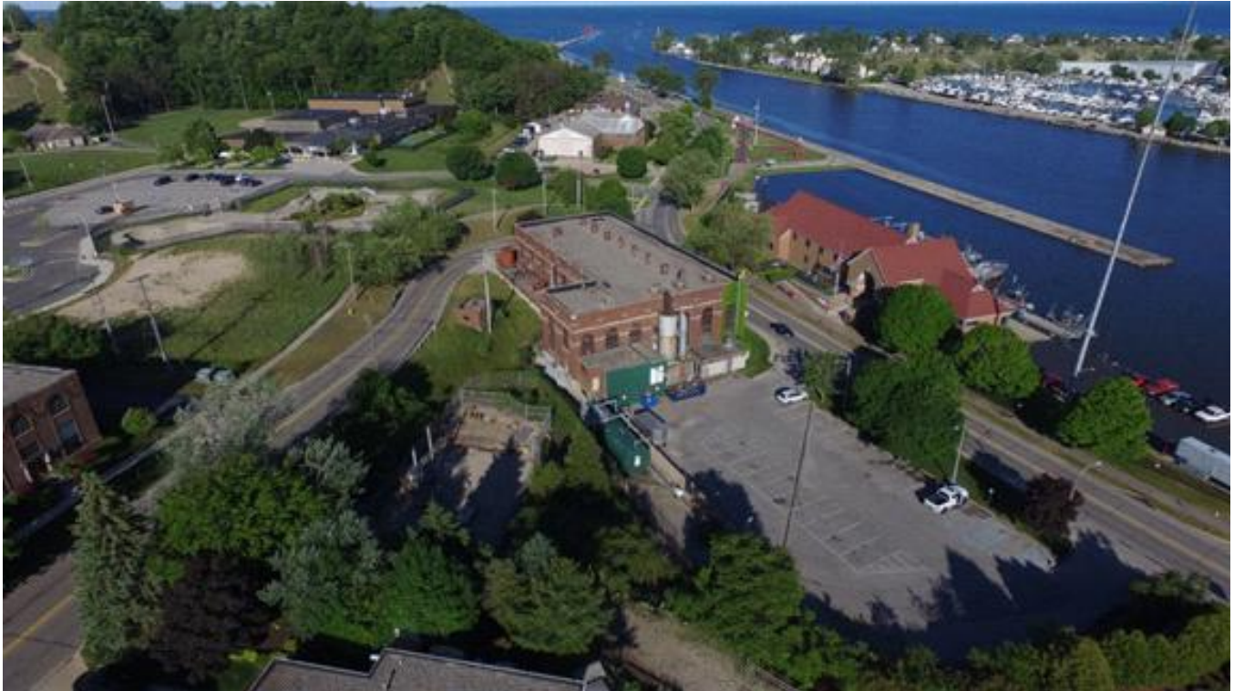
View of BLP Diesel Plant in the context of the Grand River, Coast Guard Station, Harbor Drive, Sherman Street, and nearby neighborhoods.
