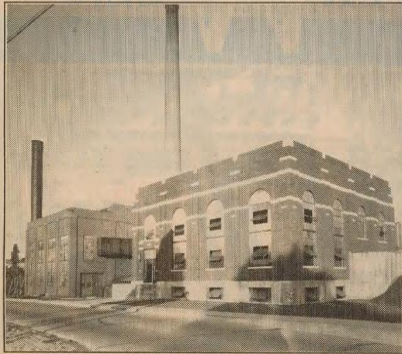
Pictured above, the original BLP generating facility on Harbor Drive, Grand Haven diesel plant (foreground) placed in operation in 1931.
