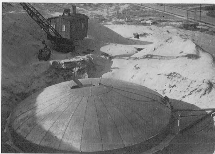
150,000 GALLON FUEL OIL TANK INSTALLATION. DURING CONSTRUCTION PERIOD.
