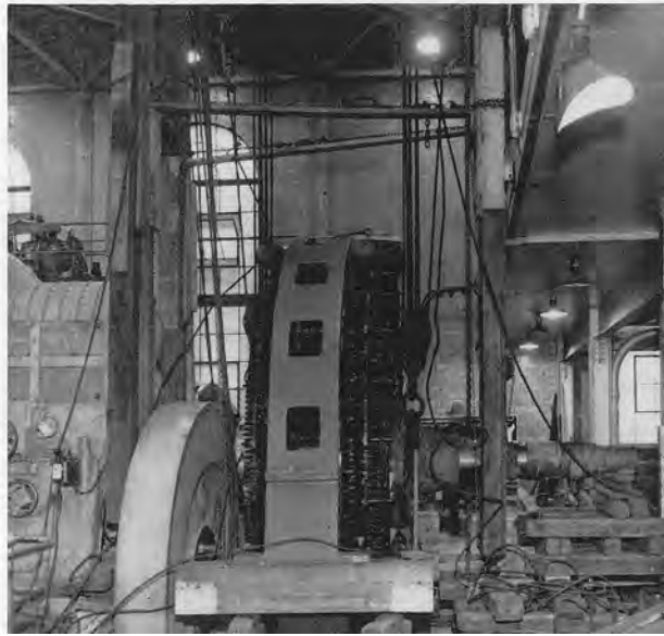
Lowering New 6900 Volt, 3390 KVA. Allis-Chalmers Generator into Position
