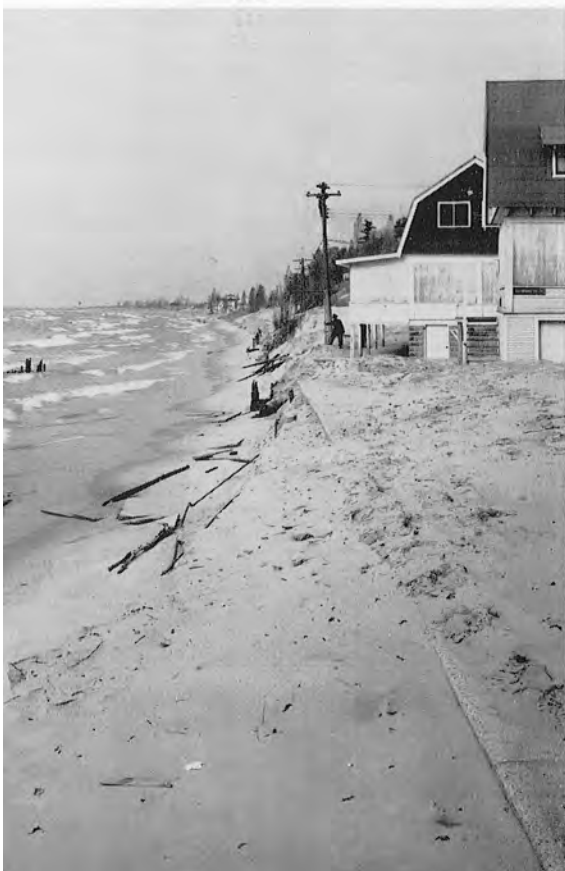
Encroachment of Lake Michigan on shore line necessitates relocating distribution lines.
