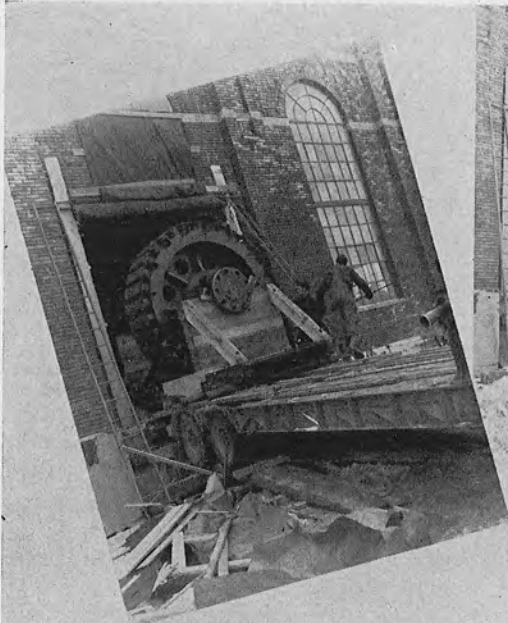
MOVING NEW 3390 KVA, 6900-7200 VOLT GENERATOR, INTO POWER PLANT.
