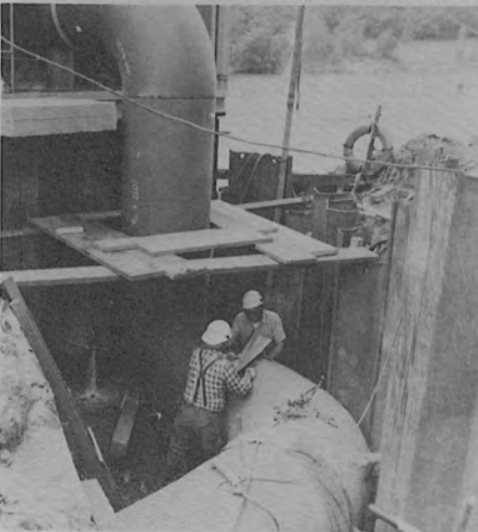
Circulating Water Discharge Pipe Installation Sims III Main Control Panel
