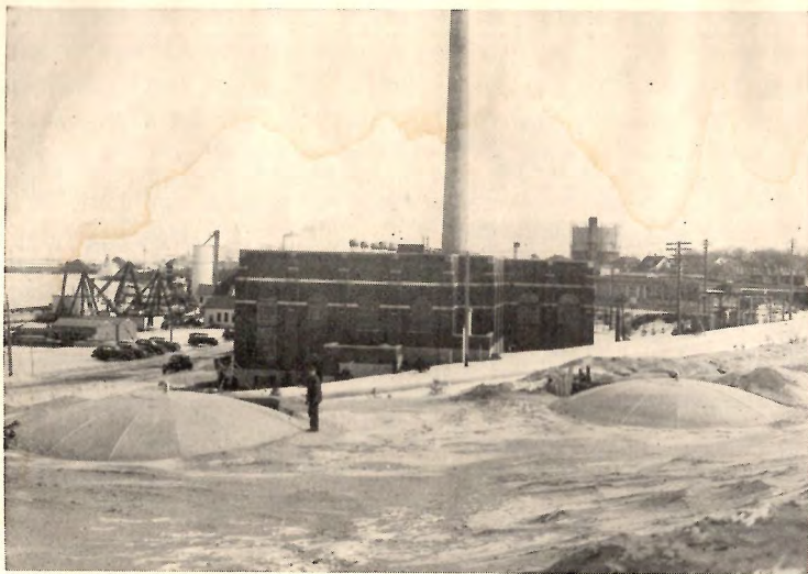
Two 100,000 gallon fuel oil storage tanks with power plant and part of harbor in distance
