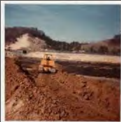
7. Spreading the initial lift of clay onto the southwest quadrant of the ash ponds.
