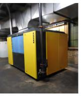
EPC improved its compressed air supply and energy consumption with installation of a Variable Speed Air Compressor in 2020 and this year replaced LED lighting.
